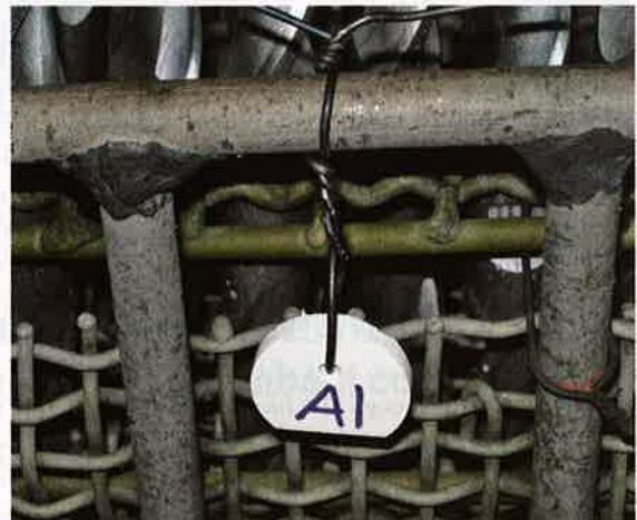
Fig. 4. TempTab wired in place during daily monitoring.
